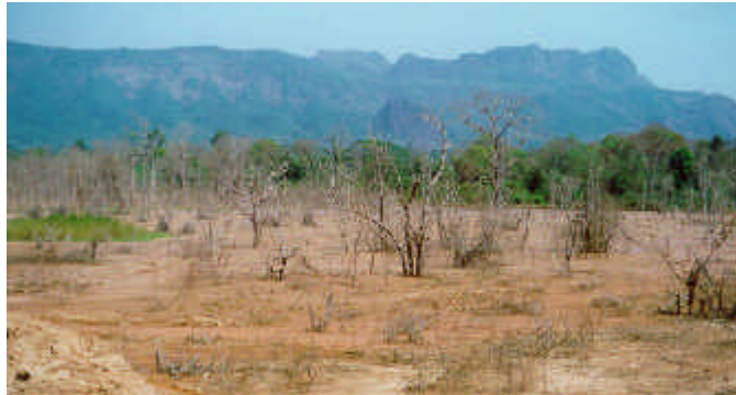
Breeched tailings impoundment at Nam Pathene Tin Mine
